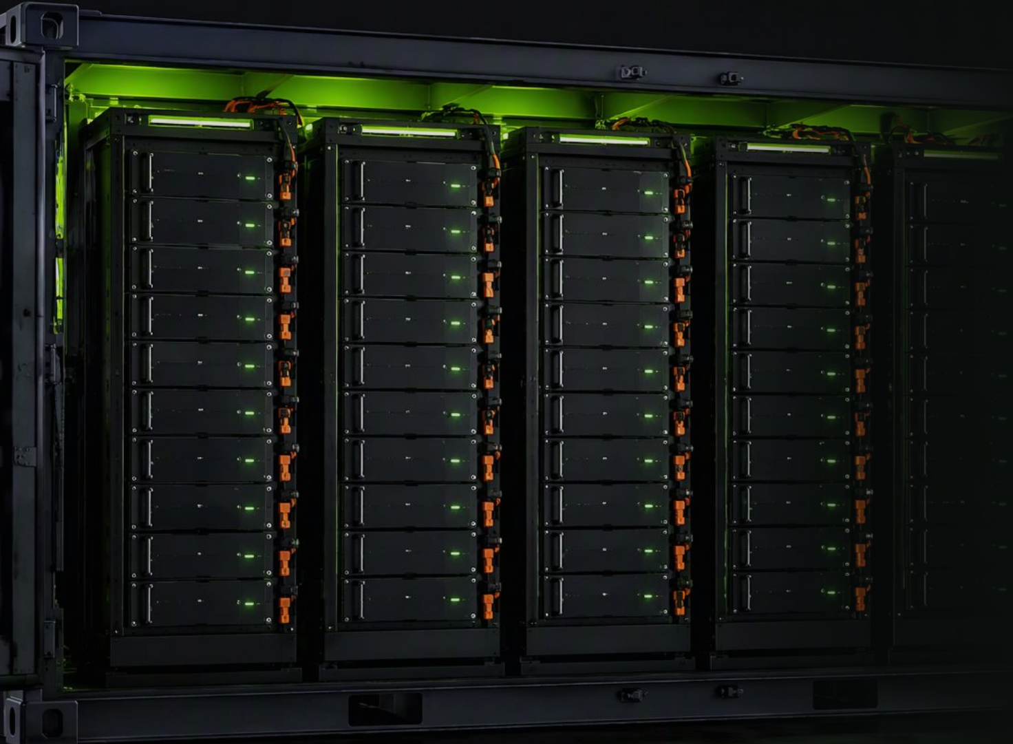
Energy365, doors open — five battery racks and the electrical compartment.
